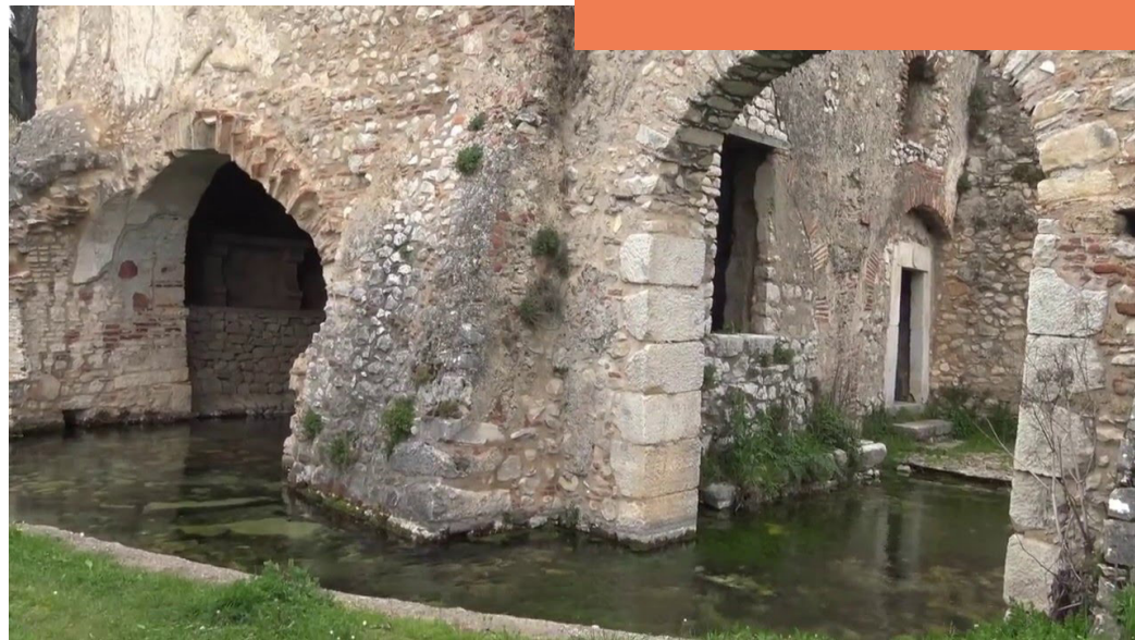
The Baptistry of San Giovanni in Fonte was built with bricks and rubble stones.
